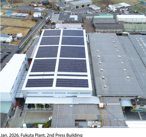
Jan. 2026, Fukuta Plant, 2nd Press Building
