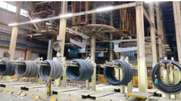
Large scale pickling line
