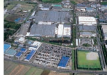
Head Office/Fukuta Plant
