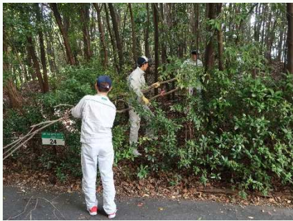
▲Cut trees are carried out
